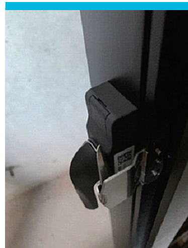
Figure 1.3.1.2-2 RFID tag attached to the frame of a window
