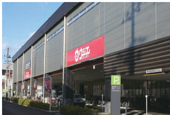
Fig. 1.1.4-3 UJIE SUPER CO., LTD Branch Store in Odawara, Miyagino Ward, Sendai City
